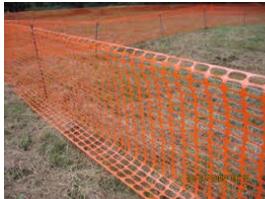
Fencing protects areas from compaction
