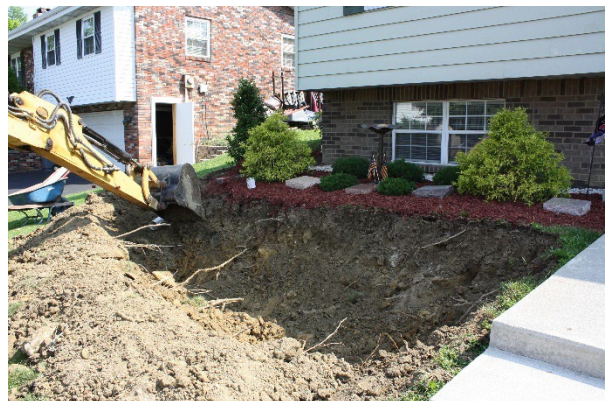
Excavate rain garden at least 10' from foundation
