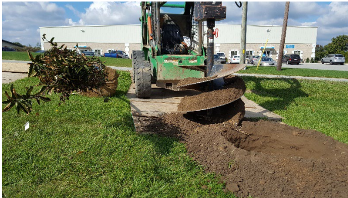
Plywood sheets protect lawn from compaction
