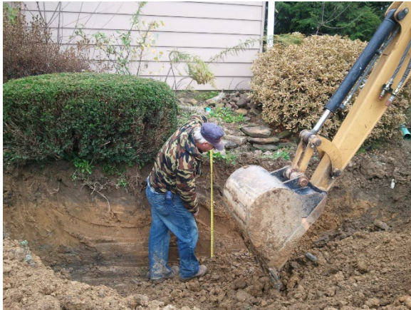
Excavate a drywell at least 10' from foundation
